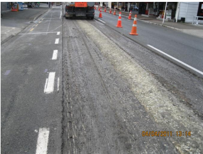
Photograph 6: Milling along SH60
