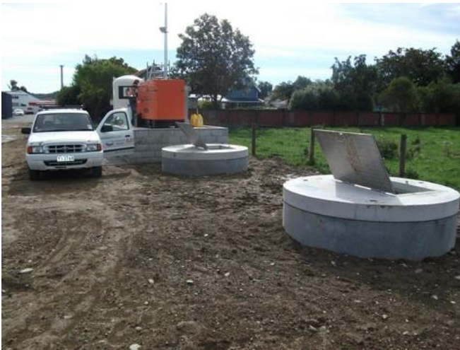
Photograph 10: Bores and generator nearing completion
