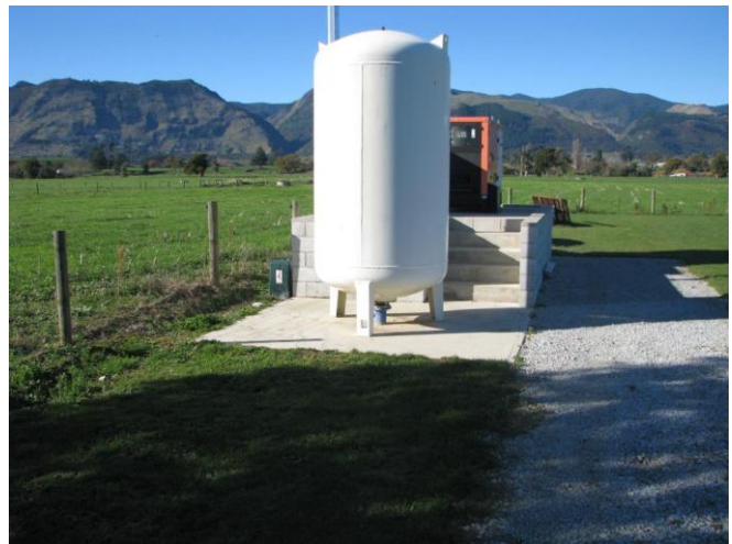
Photograph 11: Installation of the pressure vessel following completion
