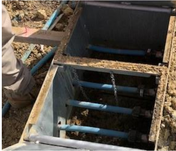
Photograph 4: Several unauthorised connections at a subdivision.
