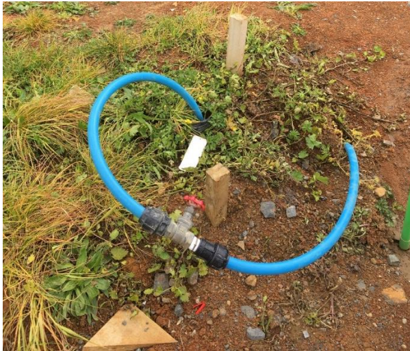
Photograph 3: An unauthorised connection at a new build.
