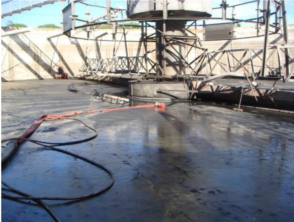
Figure 5: Clean Out of Clarifier 2
