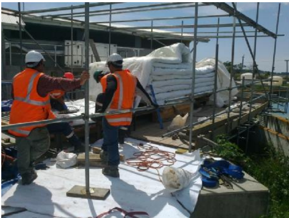
Figure 10: CIPP Liner Prior to Installation
