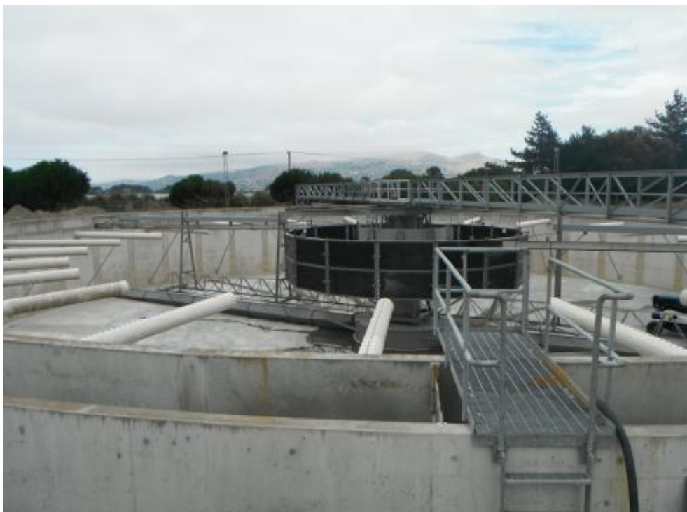
Figure 13: Fully repaired Clarifier 4
