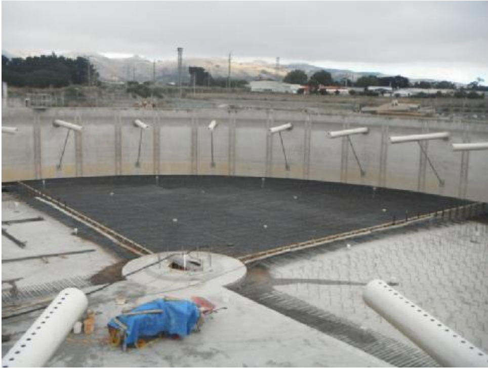
Figure 12: Clarifier 3 repairs showing reinforcing mats
