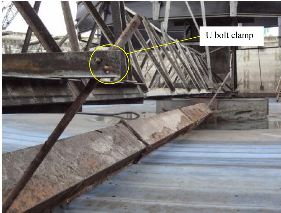
Figure 6: U-bolt scraper support
