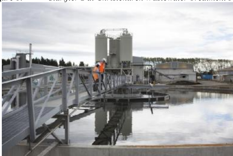
Figure 1: Clarifier 2 at Christchurch Wastewater Treatment Plant
