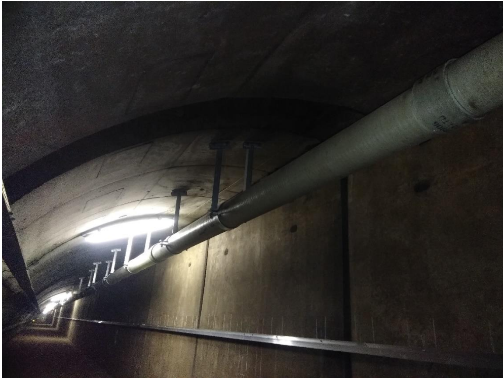
Photograph 8: DN250 GRP Pipeline Installed inside the Lyttelton Tunnel
