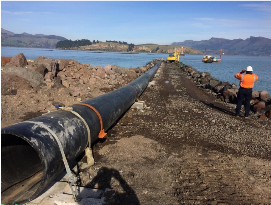
Photograph 1: Launch of Governor Bay Submarine Pipeline
