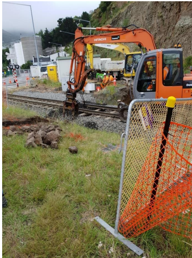
Photograph 4: Construction of pipeline under KiwiRail tracks
