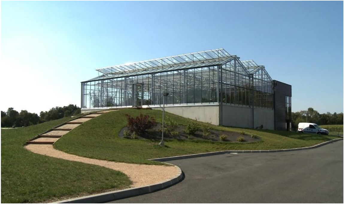
Figure 3: Le Lude STP – France. A view of the integrated process
