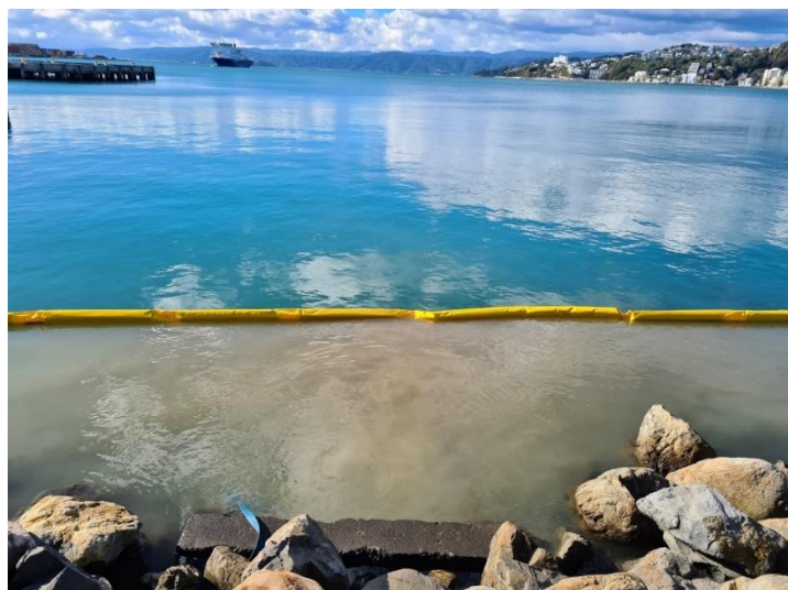
Photograph 3: Marine sediment boom (Credit: ECS / Peter Mumm)
