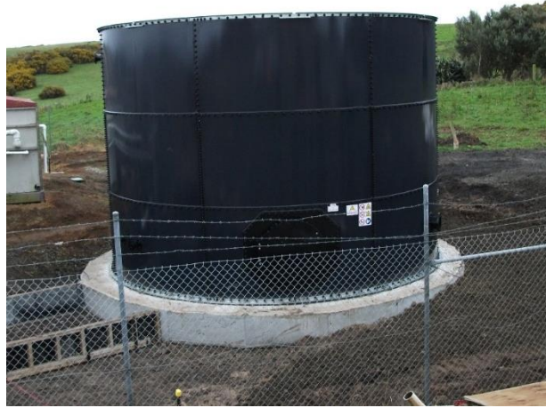
Figure 7: Newly constructed Balance Tank
