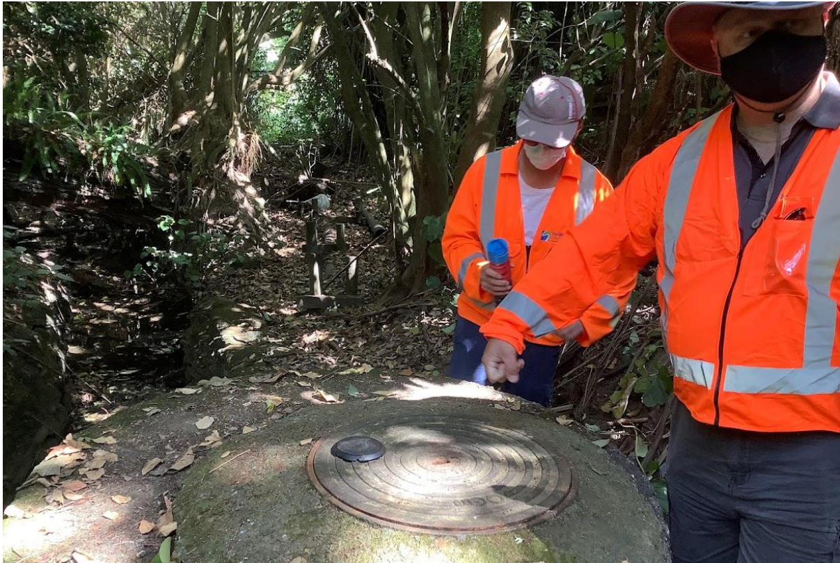
Figure 6: Manhole with sensor installed and staff preparing to mark manhole alignment. Note uneven terrain and dense vegetation in the background.
