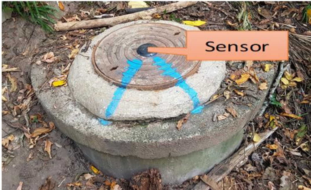
Figure 13: Image sent to contractors to explain sensors and to request the correct alignment is maintained
