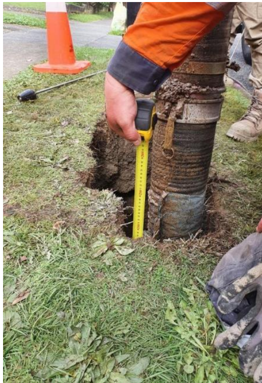
Figure 8: Typical inspection shaft being hydro excavated and finished with cover (courtesy Intergroup and Wellington Water)
