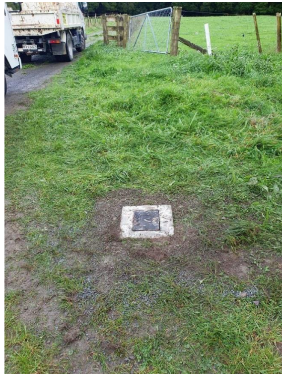
Figure 8: Typical inspection shaft being hydro excavated and finished with cover (courtesy Intergroup and Wellington Water)
