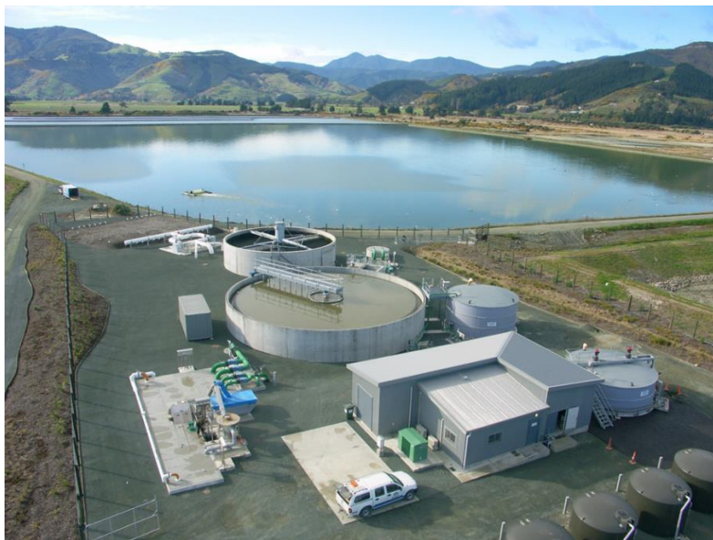
Photograph 1: Oblique view of NWWTP with land-based plant in foreground and facultative pond in background. (Source Nelson City Council).
