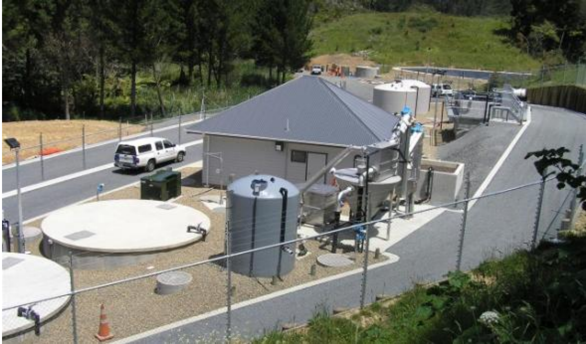
Photograph 7: Inlet Works area
