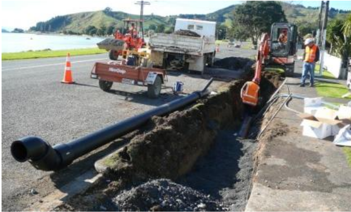
Photograph 4: No trenches exceeded 1.8m depth along the 4km of shoreline
