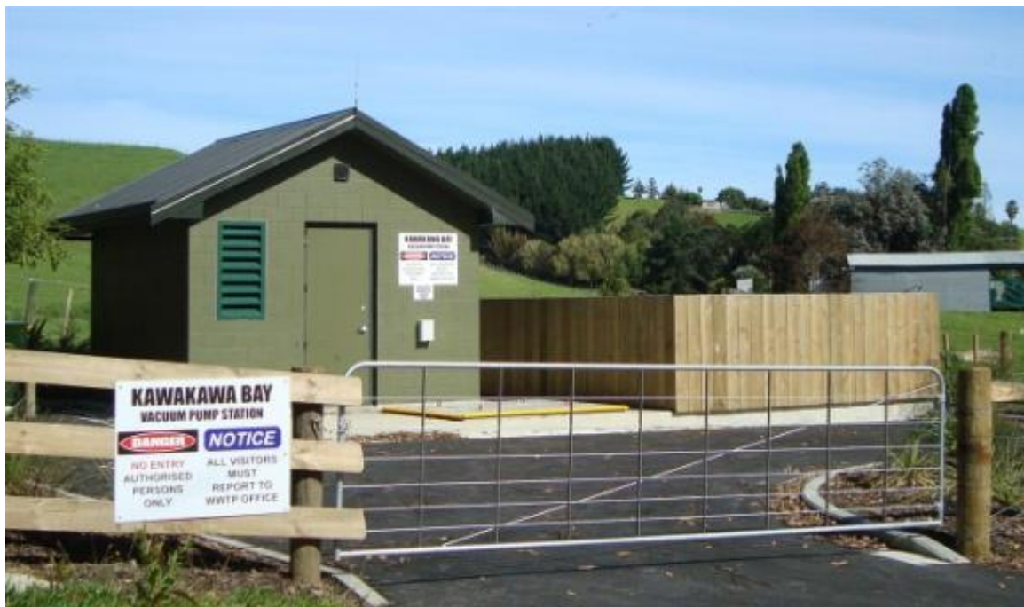
Photograph 5: Access building for the completed vacuum pumping station and biofilter
