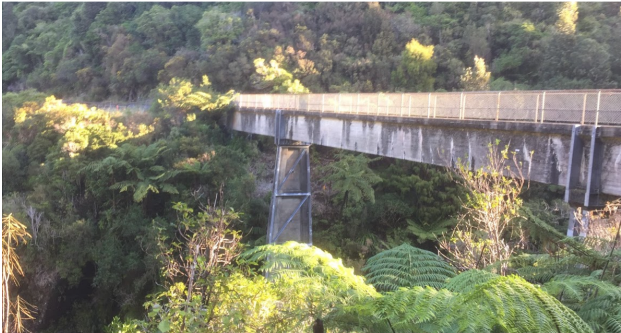
Figure 1 Existing Kaitoke Flume Bridge
