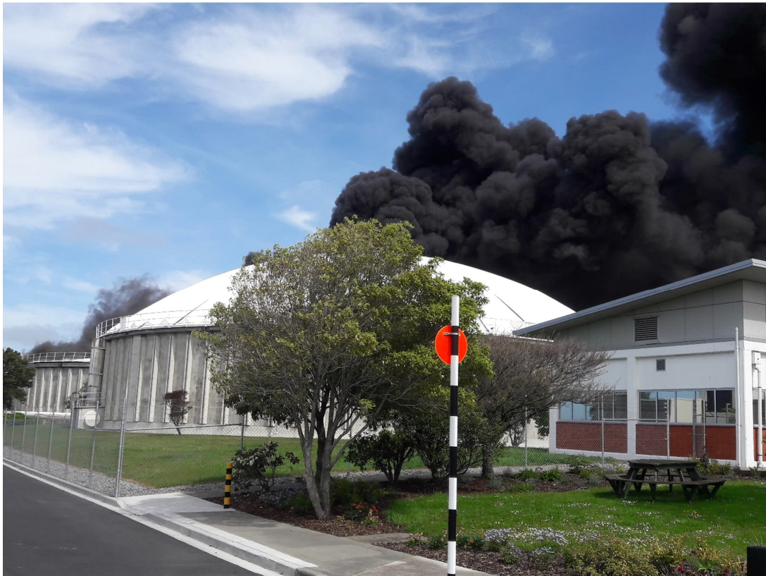
Figure 1: Trickling filters during the fire event
