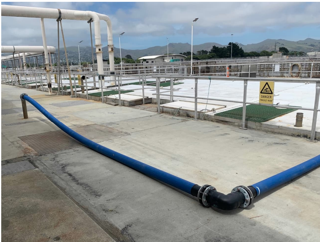
Figure 6: temporary connection from the gravity belt thickeners to the belt presses
