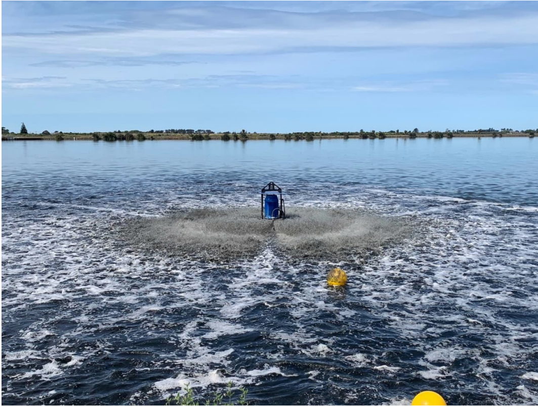
Figure 10: The aspirating aerator from Takaka
