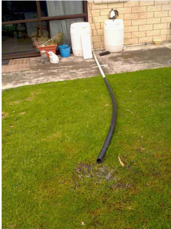
Photograph 1. Unregulated greywater disposal from a washing machine outlet onto a lawned area.
