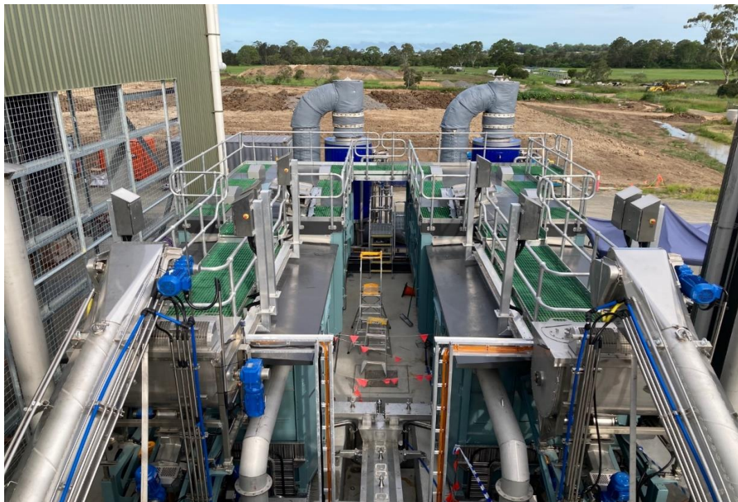
Figure 6-Picture of the Loganholme full-scale biosolid gasification plant during construction
