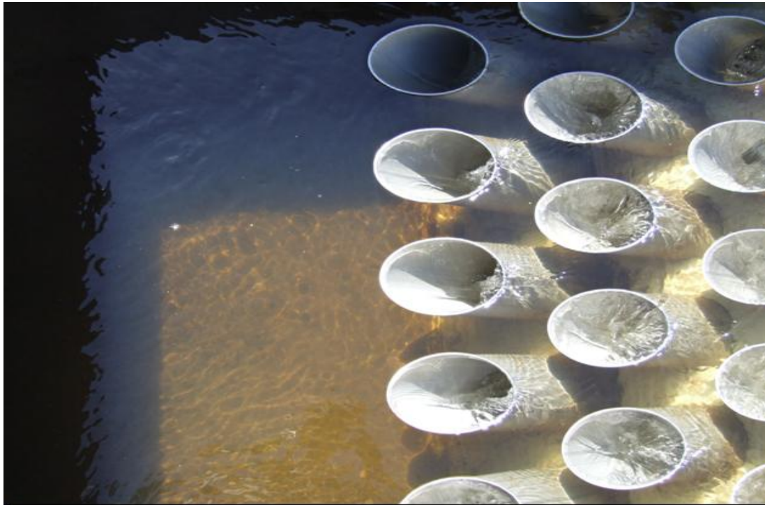
Figure 2: Treated wastewater prior to discharge to outfall
