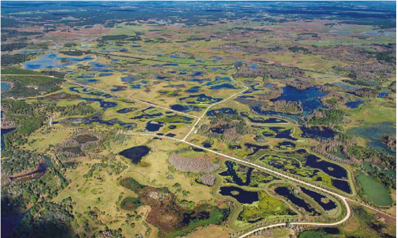
The 4G Wetlands comprises 176 acres of created wetland habitat. Located on the 4G Ranch, near Tampa, Florida, it takes excess reclaimed water from five wastewater treatment plants.
