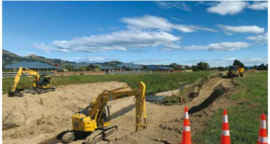
Cut-to-waste materials were transferred across the stream to allow the walkway to remain open.
