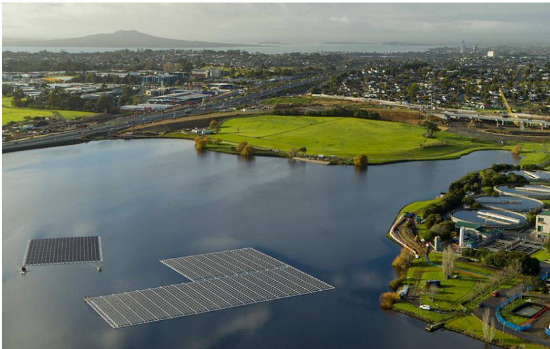
Rosedale WWTP 1,040kW floating array
