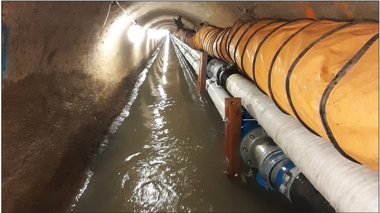
Figure 11: Over pumping set up
