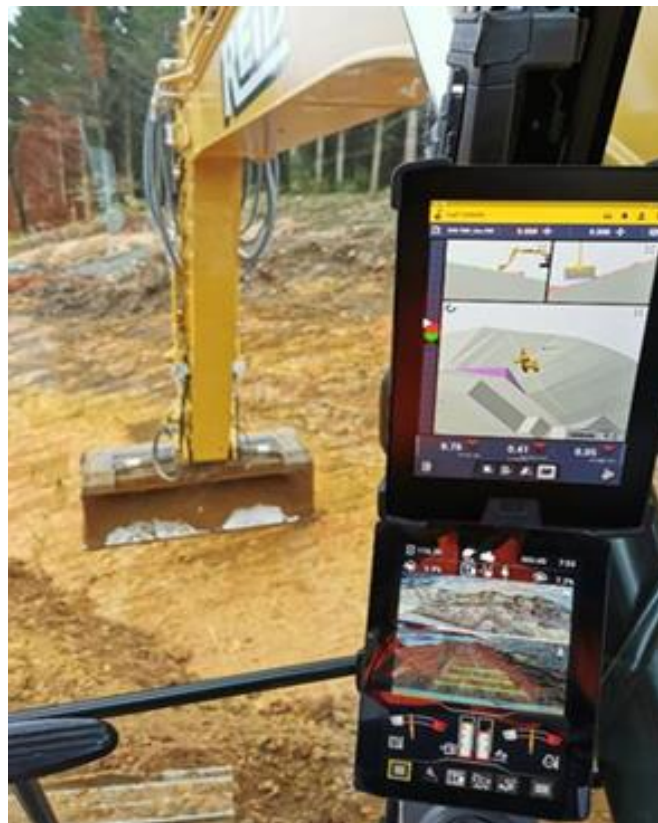
Photograph 4: "Earthwork Via Machine Controls"
