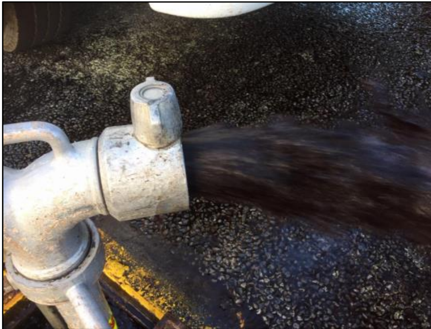
Photograph 2: Manganese Oxide contaminated pipe flush
