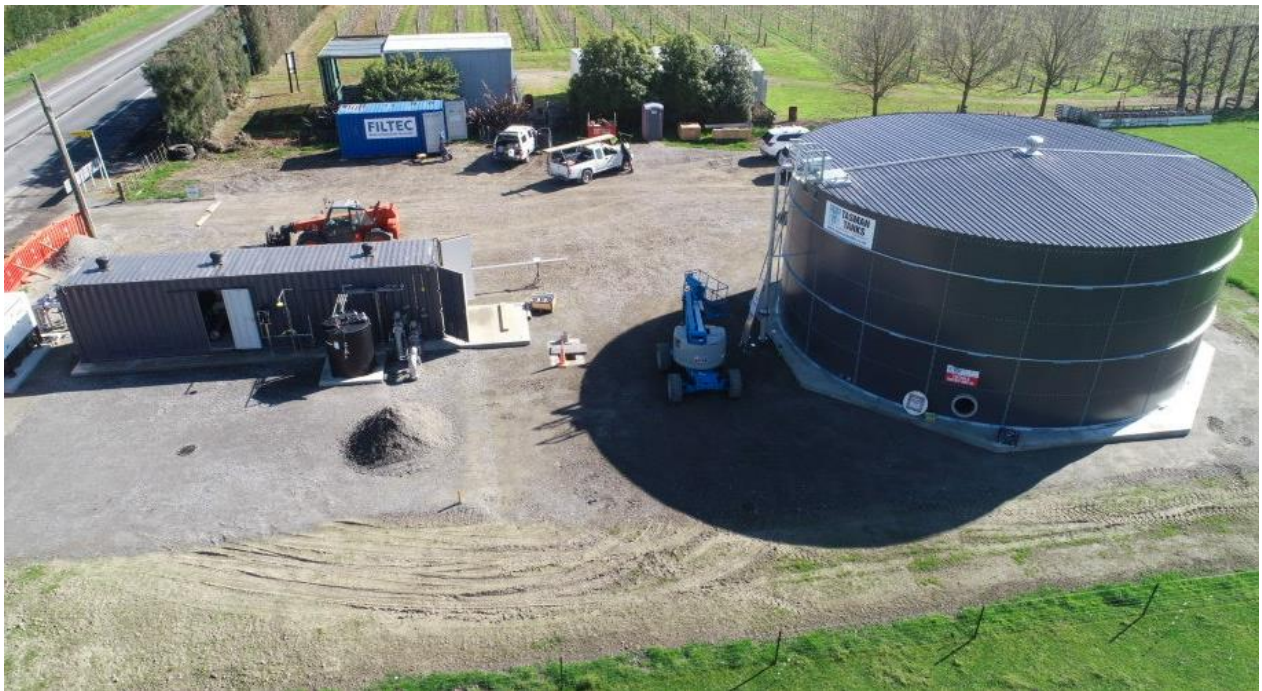
Figure 5: Hastings Small Communities: Haumoana WTP during site install.
