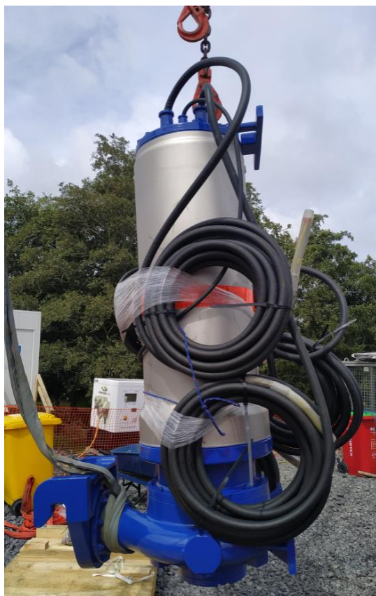
Photograph 1- Pump lift to verify centre of gravity
