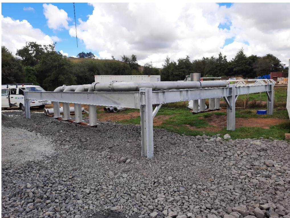
Photograph 16 - Preassembled upper half of steel frame with piping
