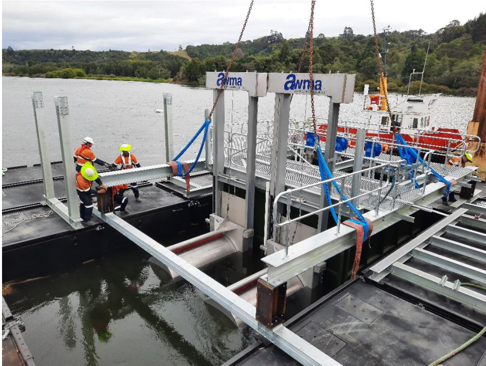
Photograph 17 - Wet well installed on temporary props
