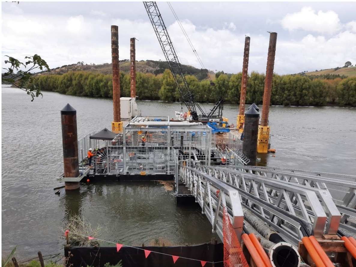
Photograph 6 - River piles and piling rig
