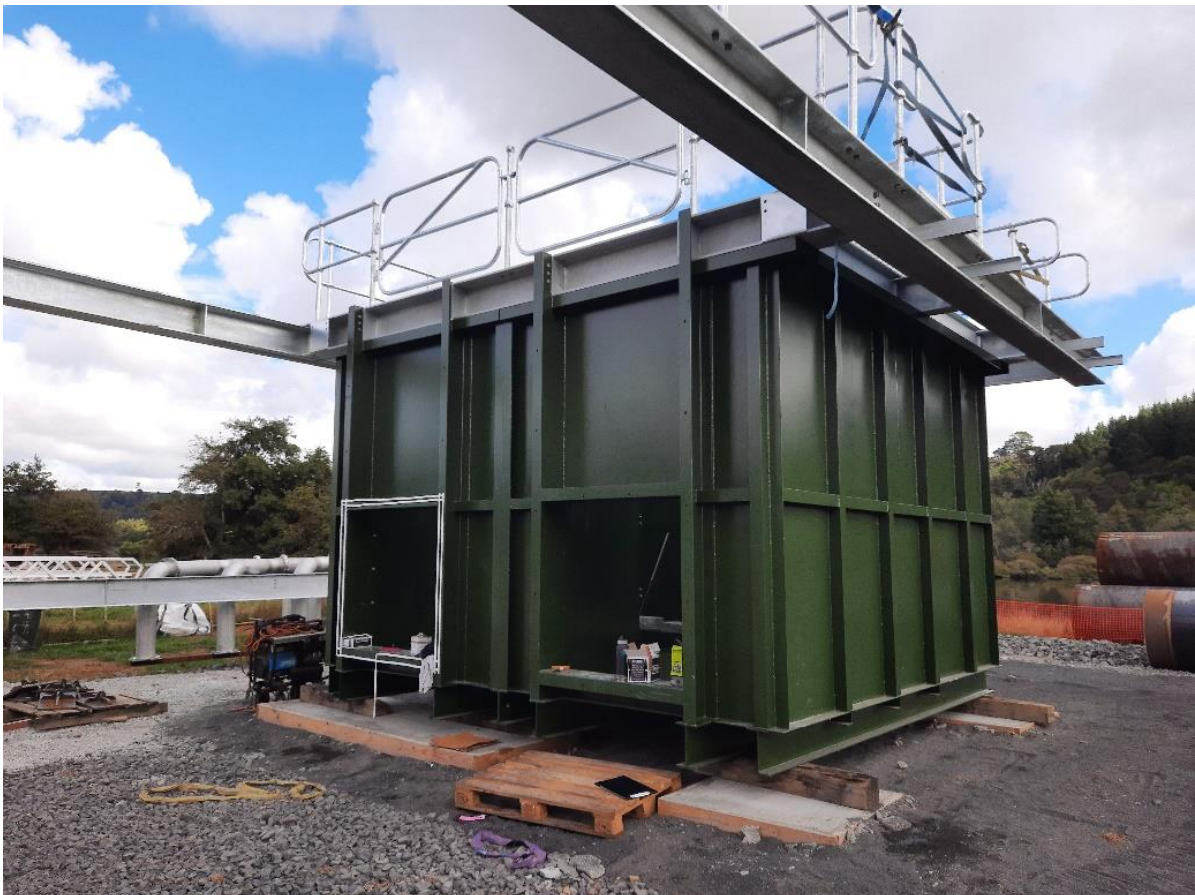
Photograph 7 - Wet well structure
