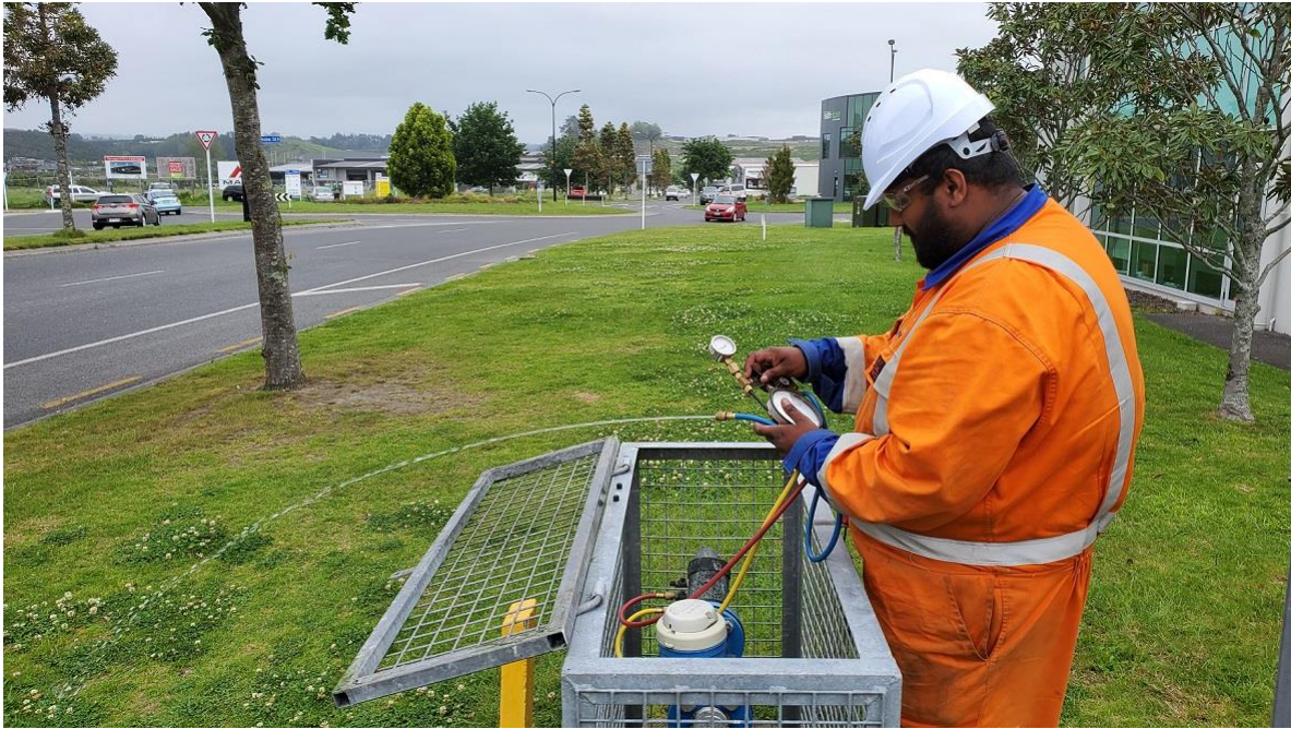
Figure 5: Nelson performing a backflow test in Tauriko
