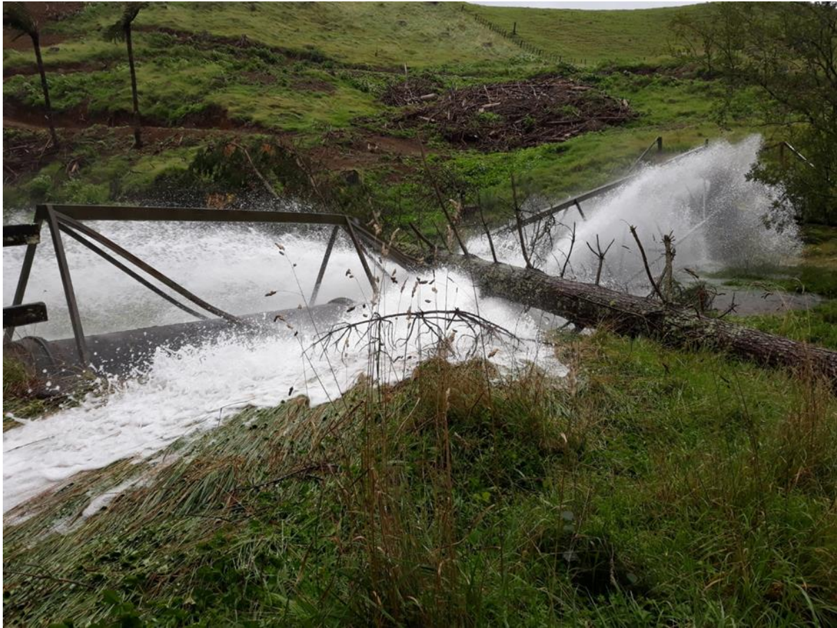
Photograph 1: Discovery of broken Pipe Bridge and water main
