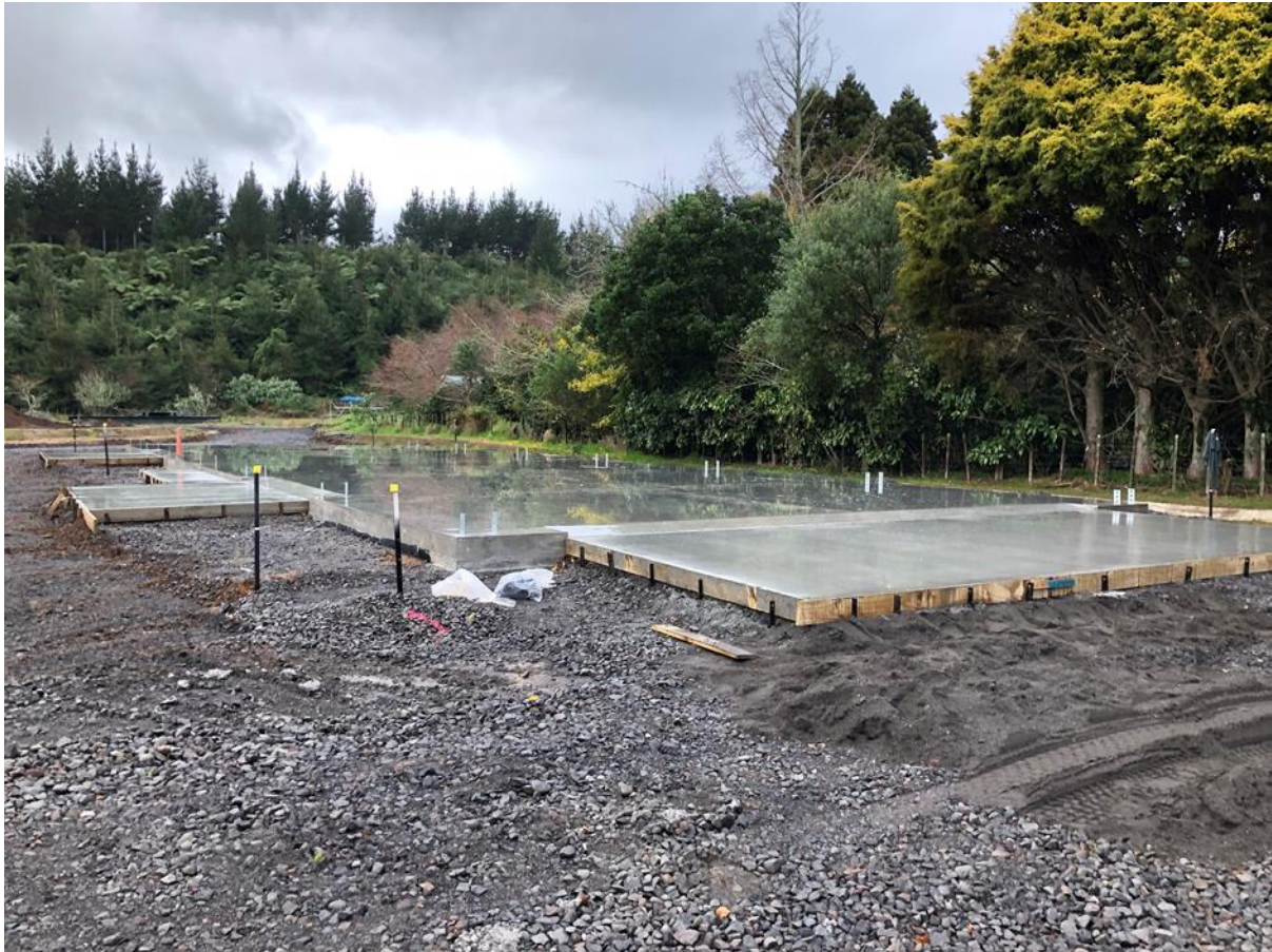
Photograph 5: New Storage Shed and Compound under construction
