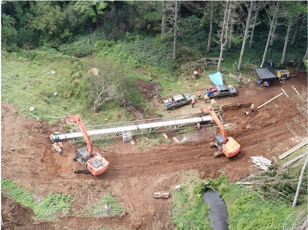
Photograph 2: Contractors repairing Pipe Bridge and water main
