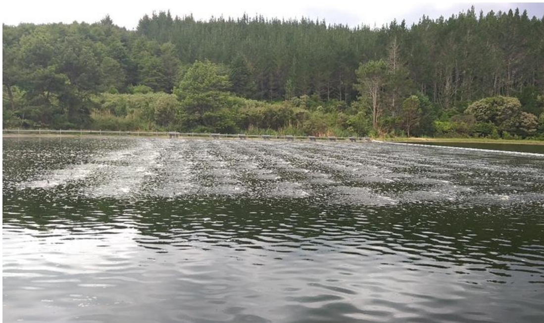
Figure 6 Bioshells® Zone showing location of Bioshells® by air pattern prior to cover installation (from Marshall Projects Ltd)
