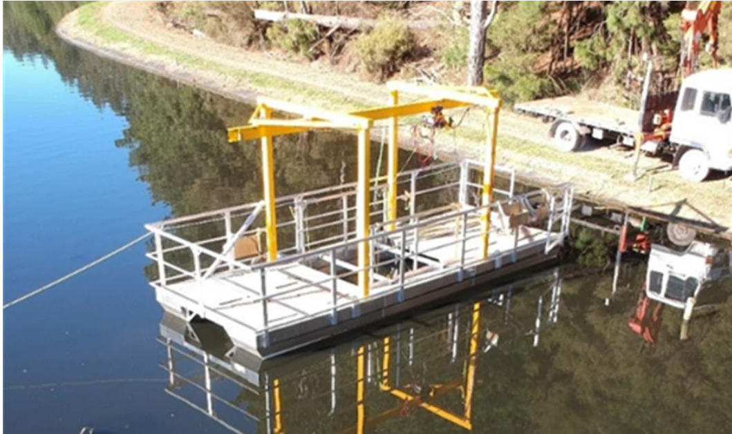
Figure 7: Innovative installation barge (from Marshall Projects Ltd)
