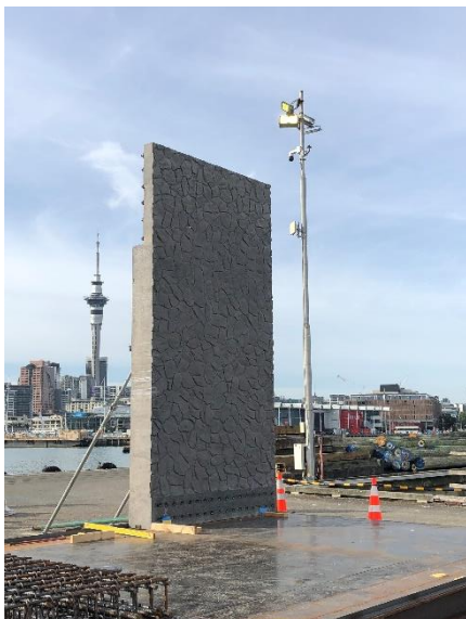
Figure 17 – pre-cast wall panels
