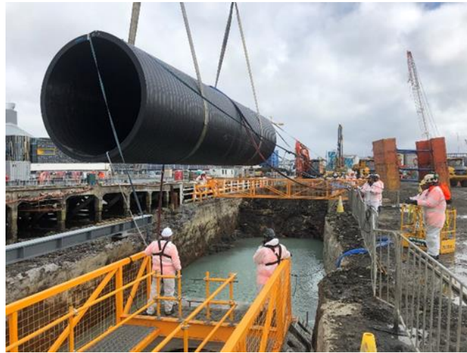
Figure 16 – HDPE pipe installation / sinking
