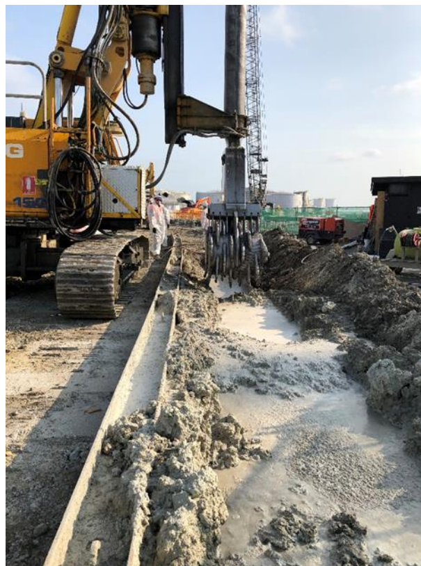
Figure 11 – CSM rig in operation
