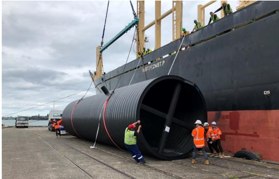
Figure 3 – HDPE pipe arrives from Thailand
