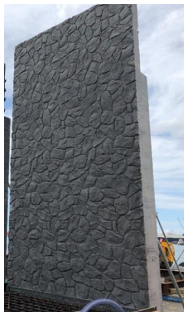
Figure 7 – patterned feature to pre-cast walls
