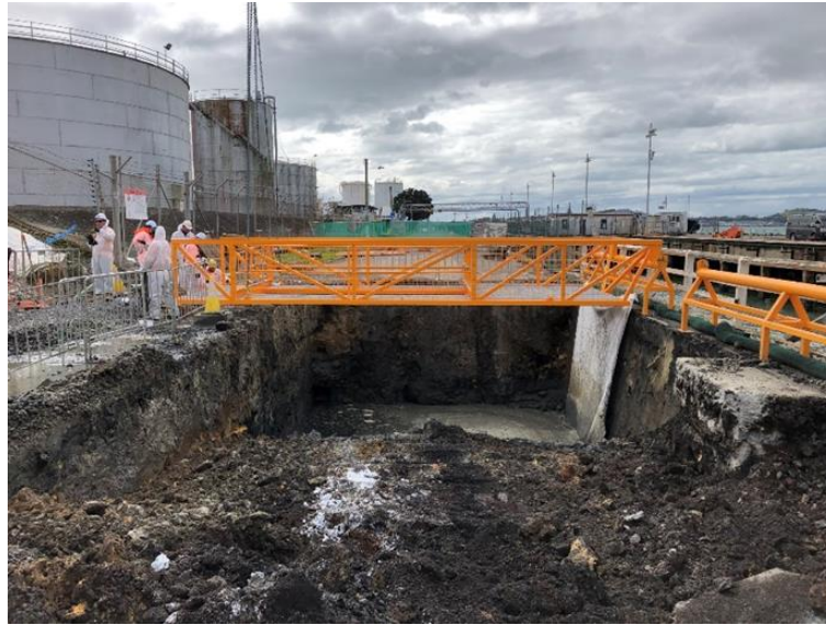
Figure 12 – steel gantry in place
