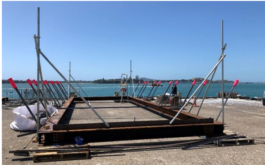
Figure 18 – headwall seating frame
