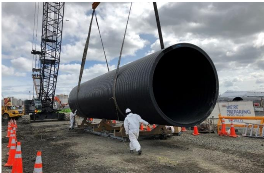
Figure 15 – preparation frame in use
