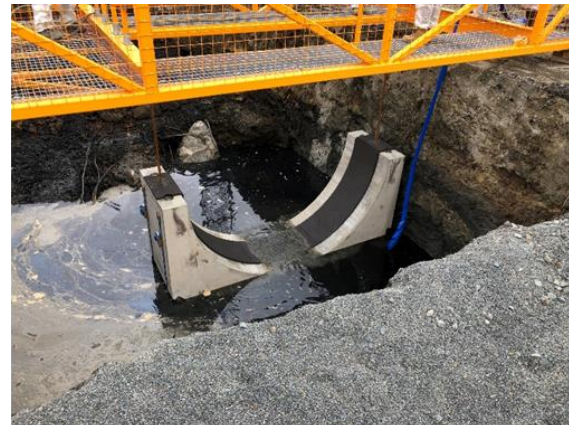
Figure 13 – installation of concrete cradle
