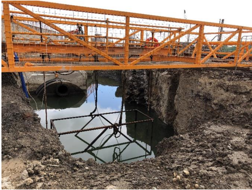
Figure 14 – survey frame in place
