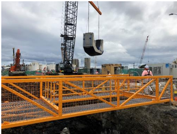
Figure 13 – installation of concrete cradle
