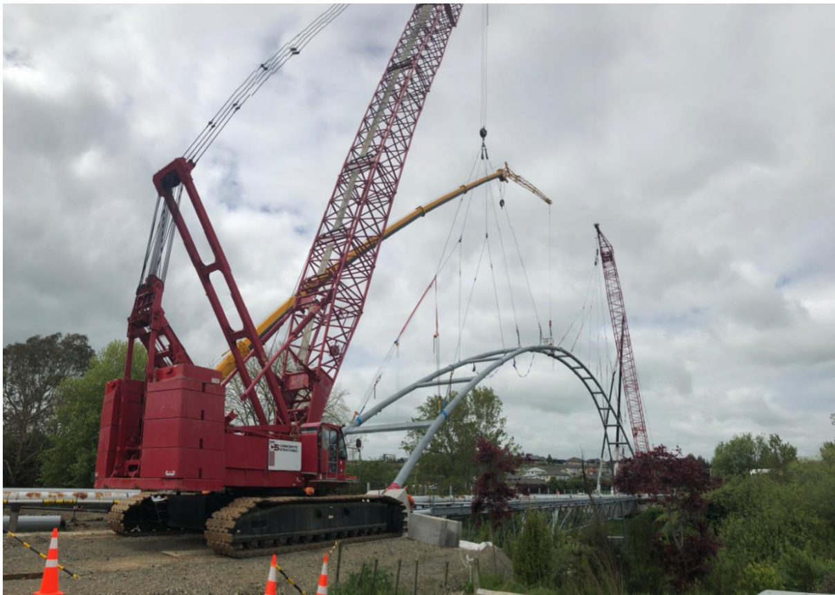
Photo 2: Network Arch Bridge Lift (October 2018)
