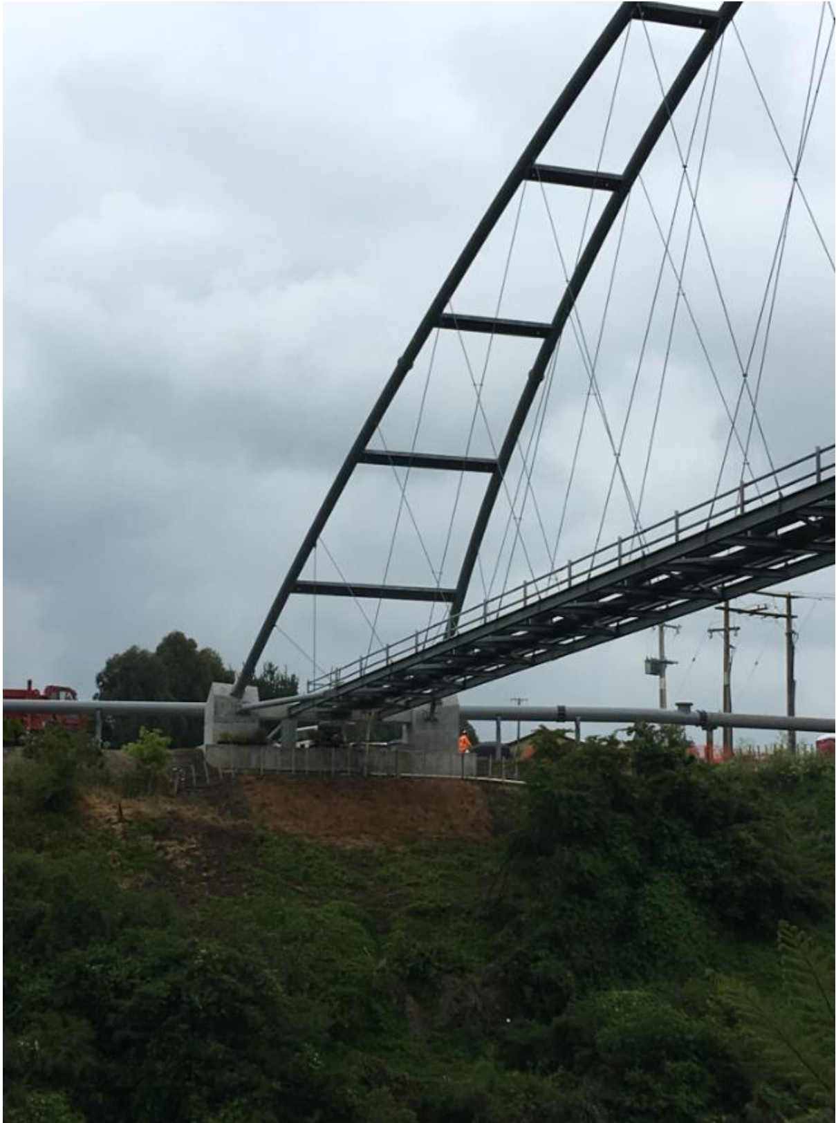
Photo 4: Completed Network Arch Bridge (December 2018)
