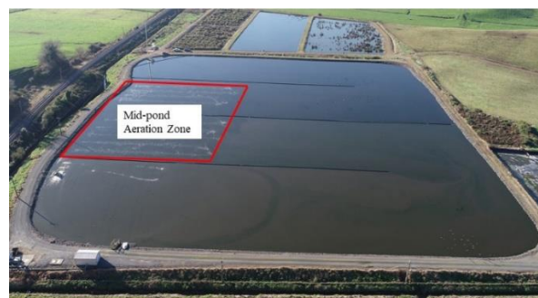
Photo 3 – Showing mid-pond aeration
