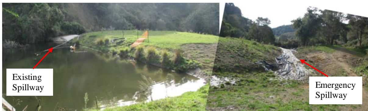
Photograph 1: The reservoir and dam crest looking toward the north, taken in 2013 before decommissioning. Note the existing concrete spillway on the left and the emergency spillway on the right.
