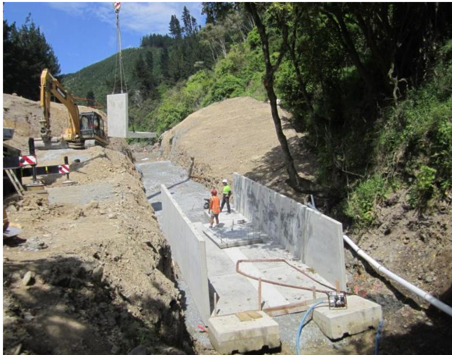
Photograph 9: installing the last of the L-Panels for the energy dissipation structure.
