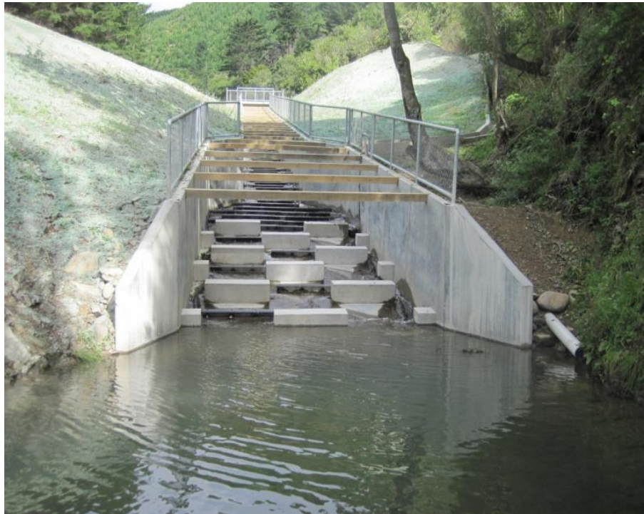
Photograph 12: Spillway with the walking track to the right and guard rails to protect the public.
