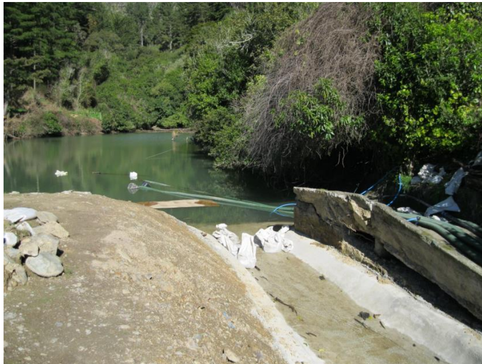
Photograph 3: Construction of the new low level spillway section.
