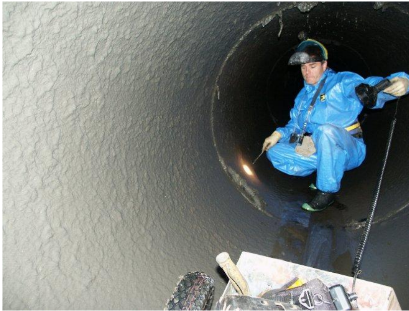
Photograph 2: Internal condition inspection 2004
