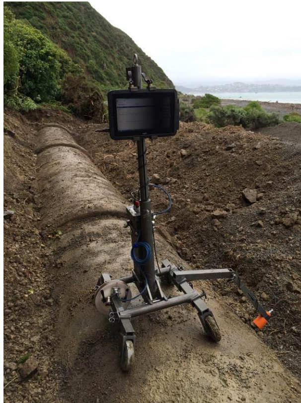
Photograph 4: External PureEM (PipeScanner)
