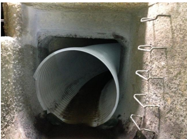
Photographs 5 & 6: Rotaloc installation in the Sewer Bend MH2-MH3
