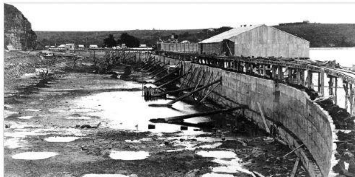
Photograph 1: Wastewater storage tanks under construction in Orakei in 1911
