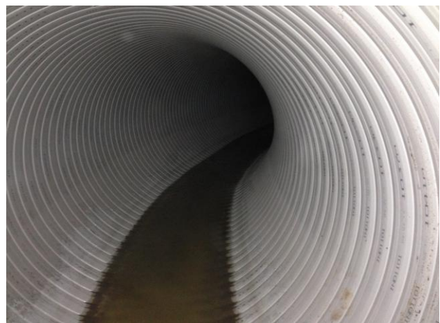
Photographs 5 & 6: Rotaloc installation in the Sewer Bend MH2-MH3
