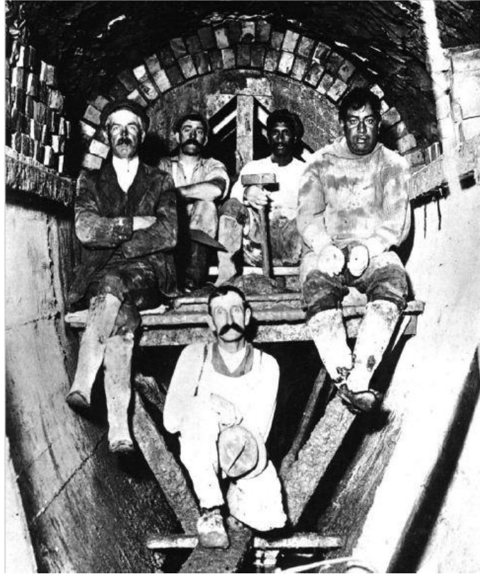
Photograph 2: Construction of the Hobson Bay Sewer
