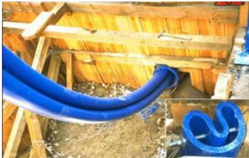
Figure 2: Fold and Form Installation
