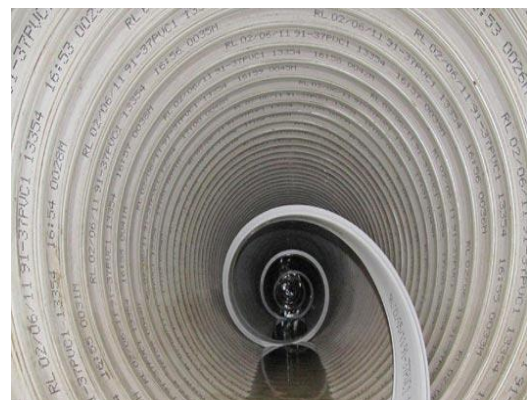
Figure 6: Spiral Wound Installation 2
