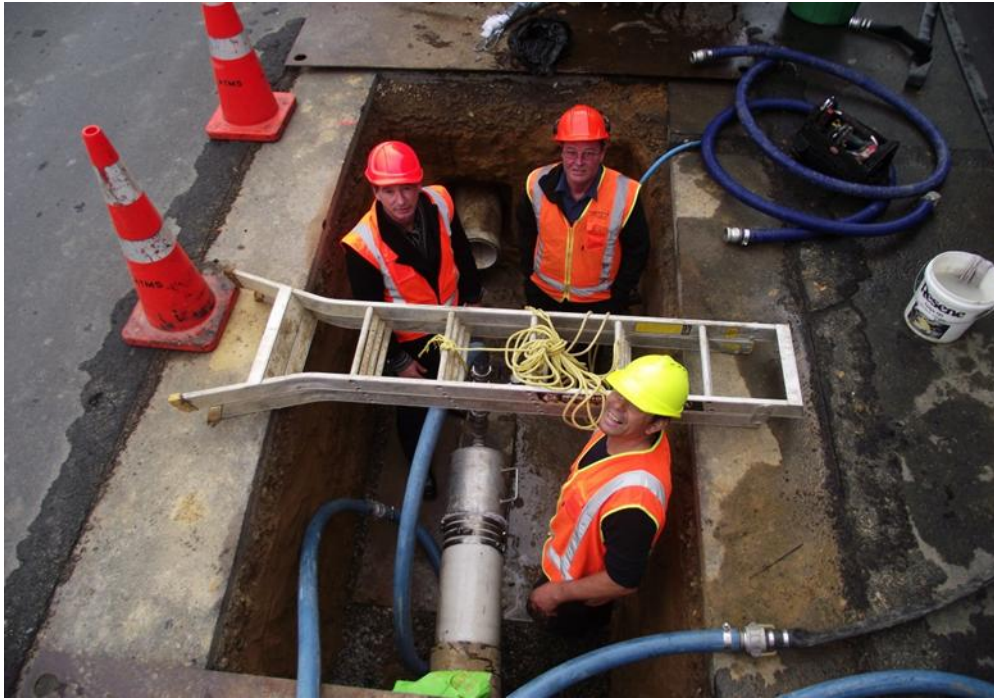
Inspection of the finished liner
