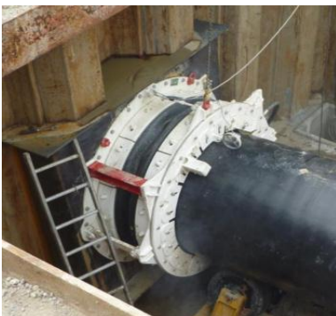
Figure 5: Direct Pipe Launch Seal
