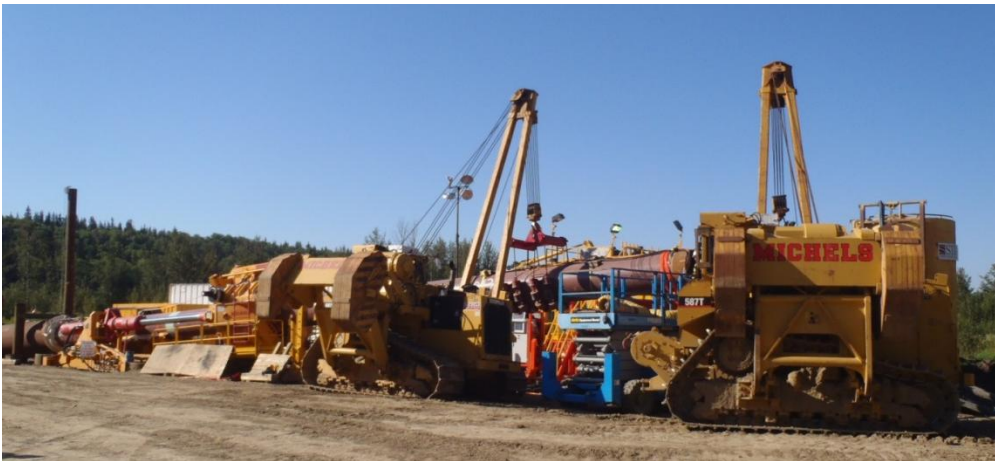
Figure 20: Side booms supporting during pipe extension
