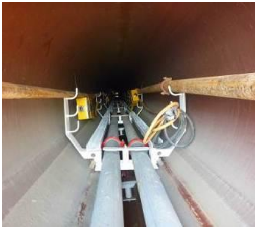
Figure 8 and 9: View into and cross-section of a 48" pipeline with supply lines placed on movable support structures
