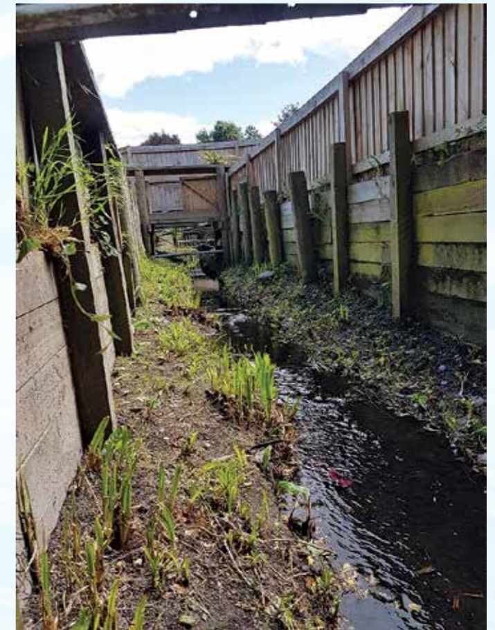
Left: The outlet to the river (no fish passage). Above: High back yard fences, vegetation and sediment build up – communities turning their back on the waterway.
