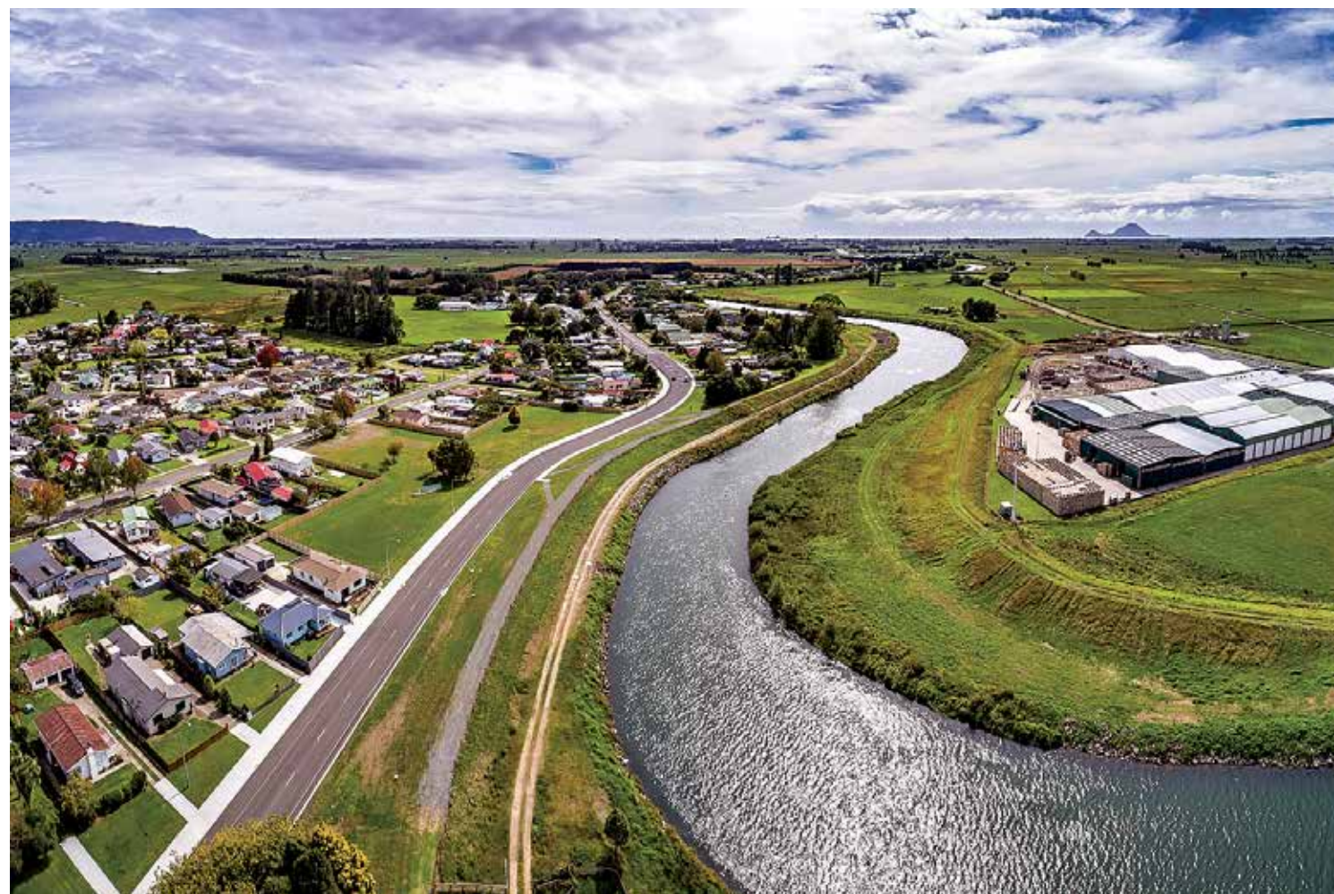
Above: Edgcumbe Stopbank completed works. The project contained three parts: excavate and remove the existing stopbank; re-build a new stopbank; and reinstate new services and build a new alignment of College Road.
