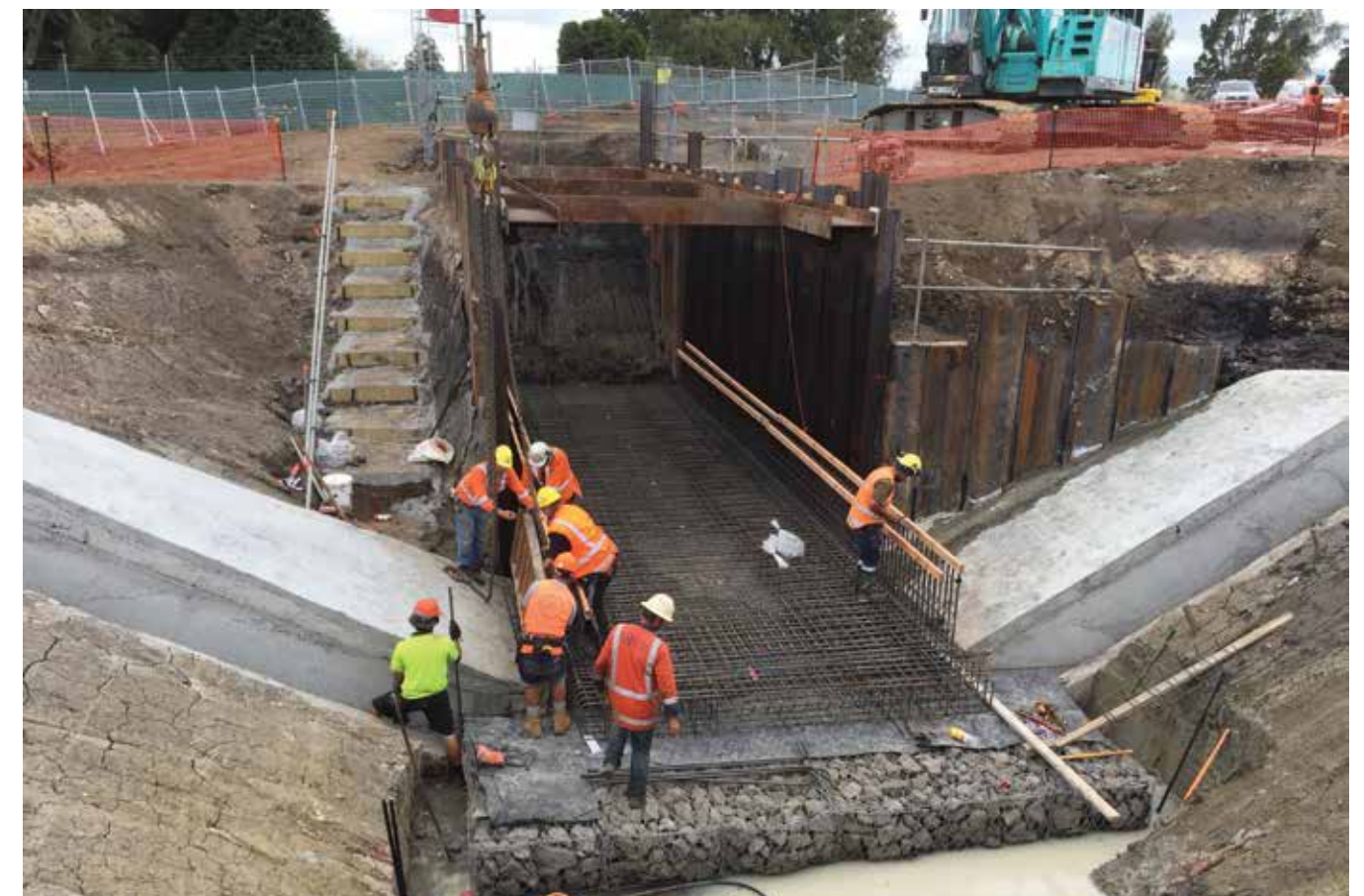
Above: Infographic representation of Takanini Integrated Stormwater Solution infrastructure upgrade project. Left: The Artillery Drive Stormwater Tunnel. Below: Construction of the Grove Road Box Culvert.
