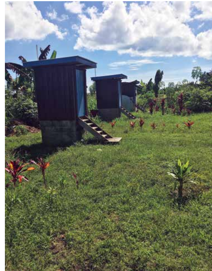
Opposite: Kiribati – the region is working towards changes but there's still a long way to go to create safe and sanitary environments for children and adults alike. Left: Raised ventilated improved pit (VIP) latrines at a school in Guadalcanal, Solomon Islands. Below: Tippy taps for improving access to hand washing facilities in Guadalcanal, Solomon Islands.
