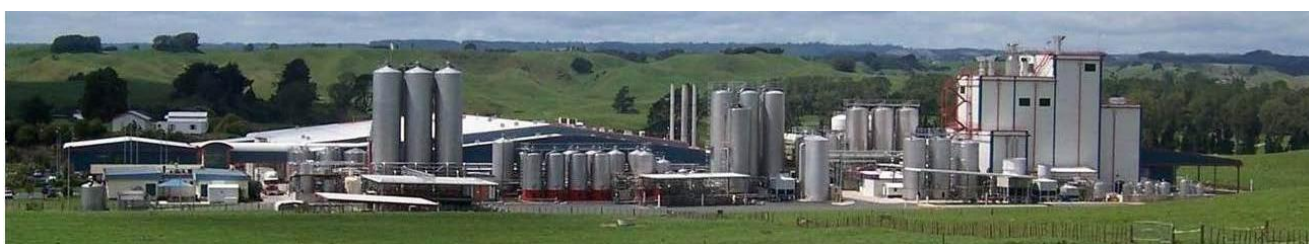
Figure 2: Fonterra Lichfield, viewed from the west, looking towards State Highway 1, prior to commencement of 2016 expansion works.
