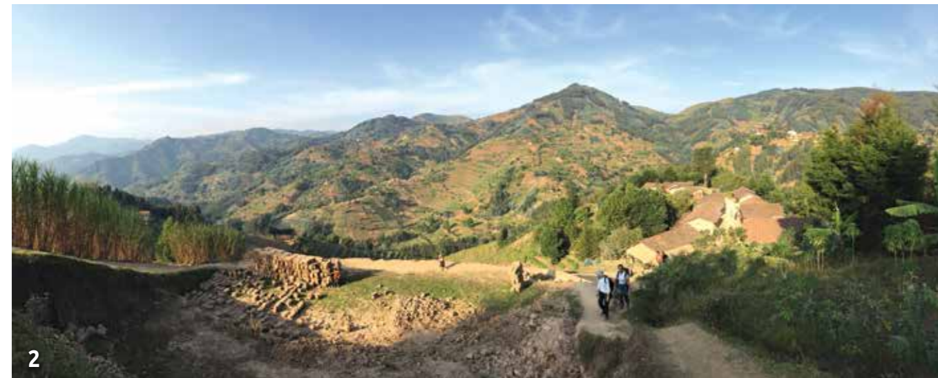
1. Previous page: The team working on one of the abutments with a line of onlooking kids watching patiently from behind the safety tape. 2. Rewarded with stunning views of the surrounding hills on our afternoon walk back up from the work site. 3. The bridge decorated in balloons ready for the official opening and ensuing celebrations.
