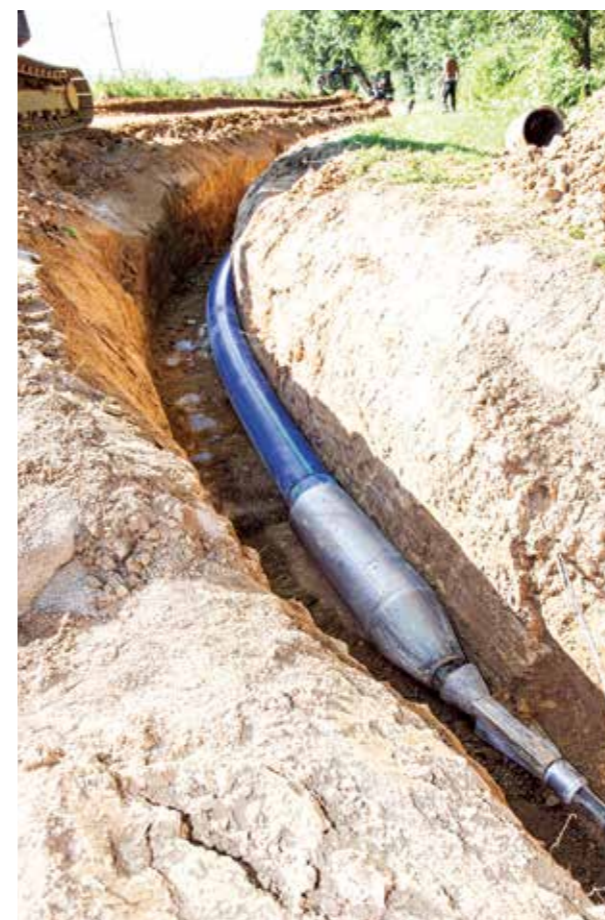
The CNC welding machine ST CNC 2. 0 supplied by AGRU ensures perfect welding seams. The bursting head and expansion cone are already mounted on the pipe. The fibre cement pipe is burst in the starting pit and a PE pipe with a larger diameter is drawn in.
