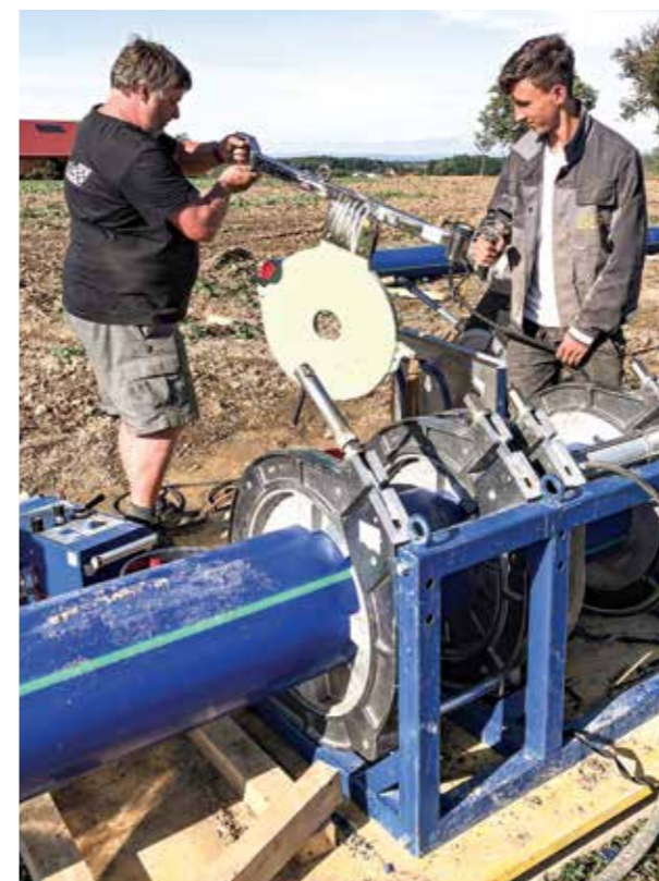
The CNC welding machine ST CNC 2. 0 supplied by AGRU ensures perfect welding seams. The bursting head and expansion cone are already mounted on the pipe. The fibre cement pipe is burst in the starting pit and a PE pipe with a larger diameter is drawn in.
