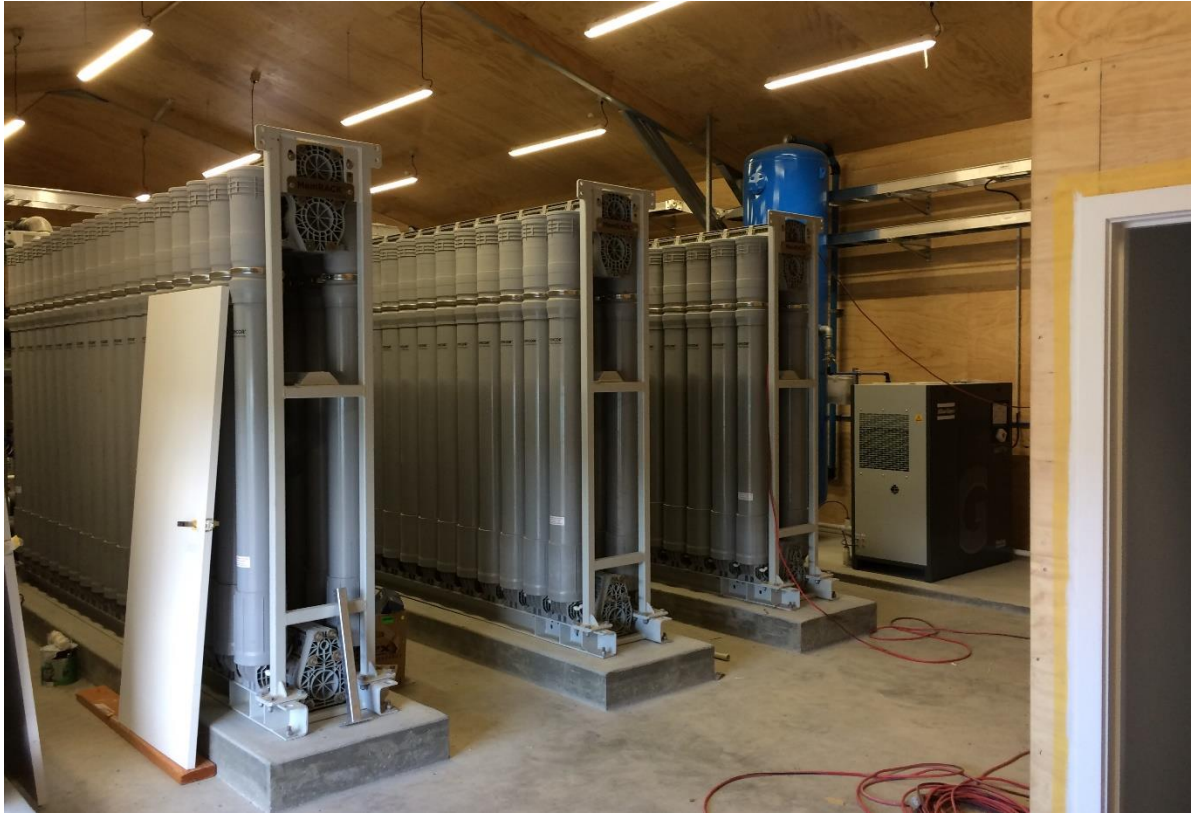
Client: Central Otago District Council Contractor: Downer NZ
