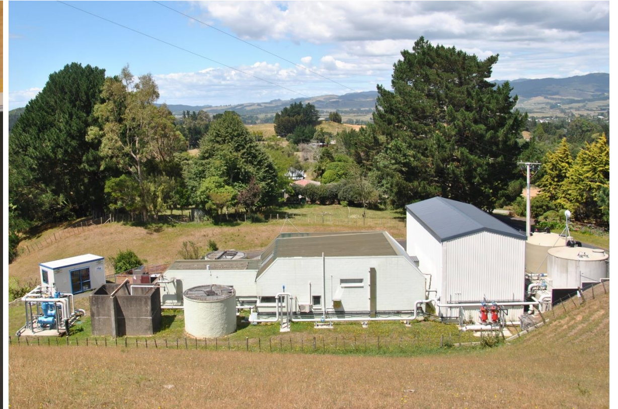
Client: Hauraki District Council Contractor: Filtec
