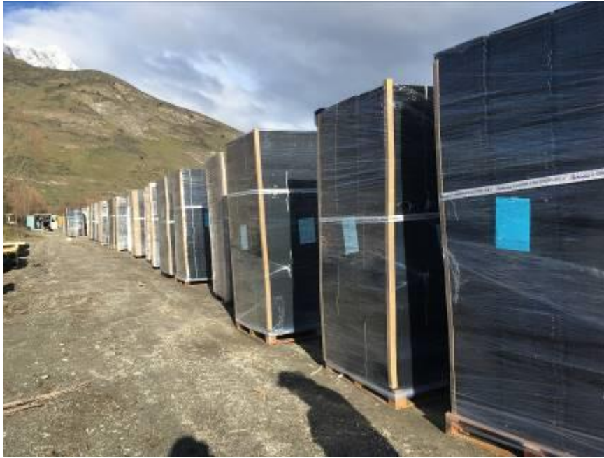
Figure 8: Water cells were delivered to site as 'flat packs', requiring assembly on site
