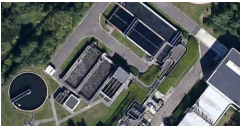
Photograph 2: Schilde conventional activated sludge lane prior to MABR upgrade
