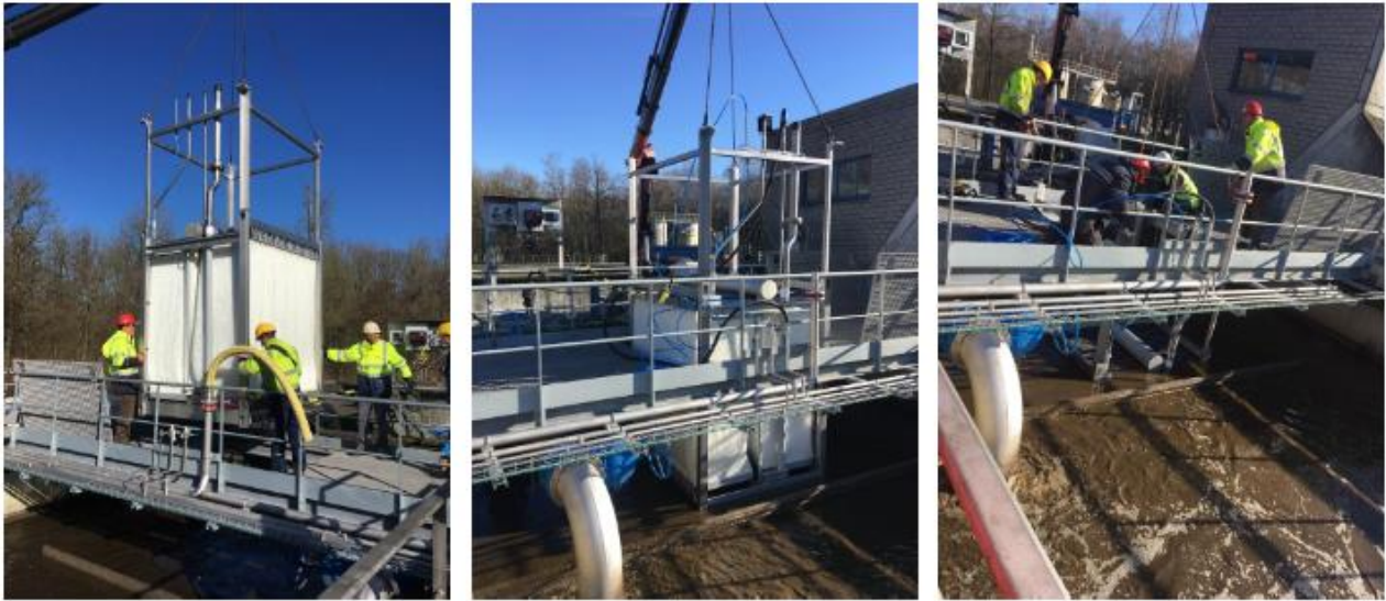
Photograph 3: ZeeLung cassette installation in existing tanks at Schilde
