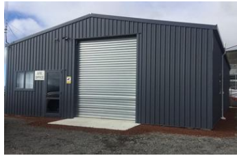
WTP Main Building
