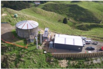
Aerial View of WTP Site
