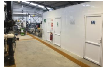
Main Corridor Inside Building
