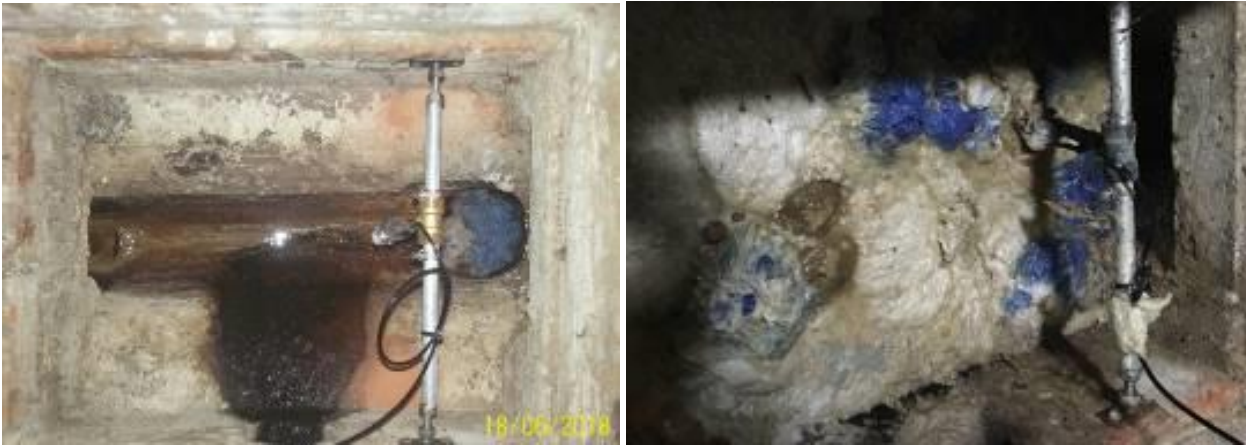
Photograph 5: Example of successful blockage location from a PLA
