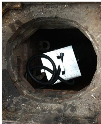
Photograph 1: An in-network dosing unit.
