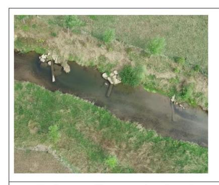
Example of a series of log groynes keyed into the bank and with additional boulder anchors (image supplied by Waikato Regional Council).
