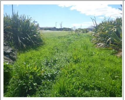
Example of a constructed stream which has approximately 0.5m of aggradation across the bed, likely due to an over-wide channel.
