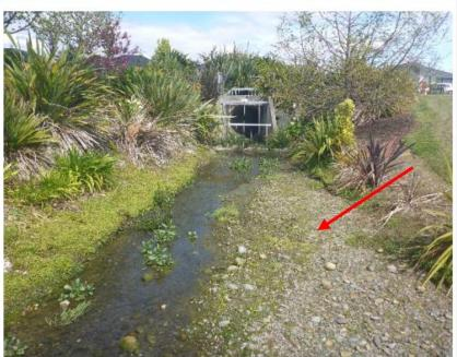
Example of a constructed stream which is over-wide and will be prone to aggradation. Note aggradation beginning to occur on the right of the photo (red arrow).
