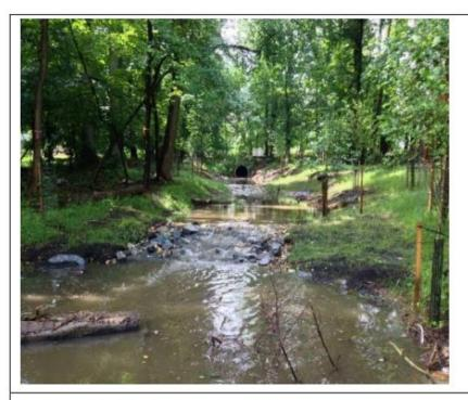
An example of a series of rock riffles fitted into a natural stream to control bed degradation (incision) (image from Department of Environmental protection Maryland, 2018).
