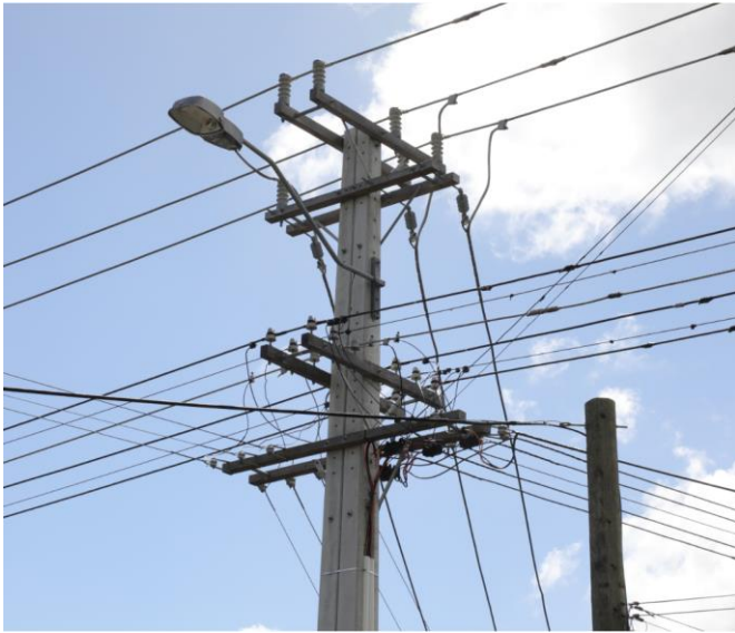
Figure 2: Distribution low voltage and medium voltage multi-circuit power lines
