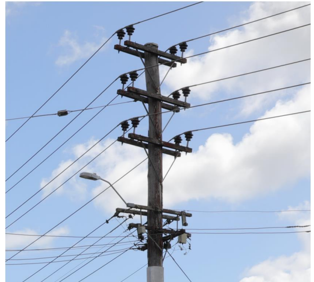
Figure 2: Distribution low voltage and medium voltage multi-circuit power lines
