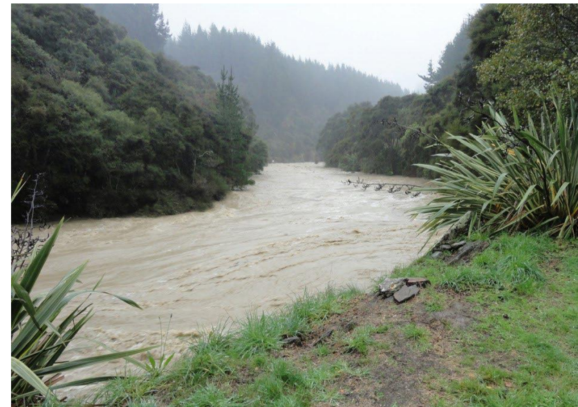
Former Herbert-Waianakarua water supply intake (Flood conditions)
