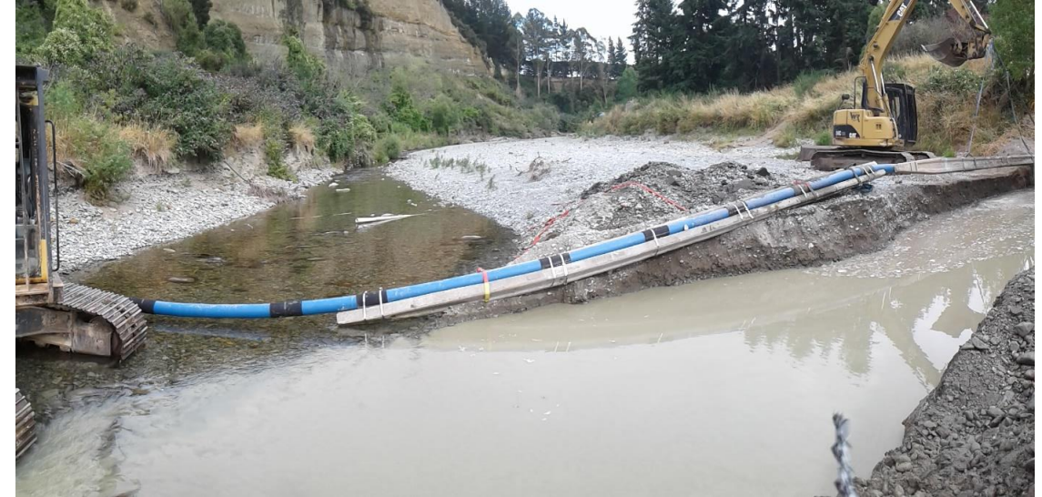
Kakanui river crossing
