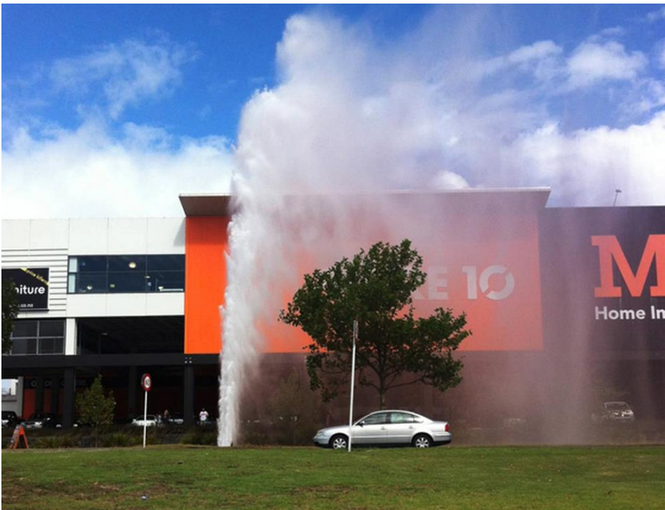
Figure 4 – Water Main Burst in Albany, 2015(Source: Stuff)
