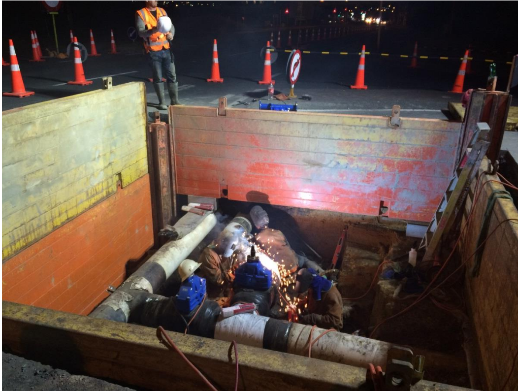
Figure 6 – Valve and hydrant installation on 300mm bulk main, Albany WSZ
