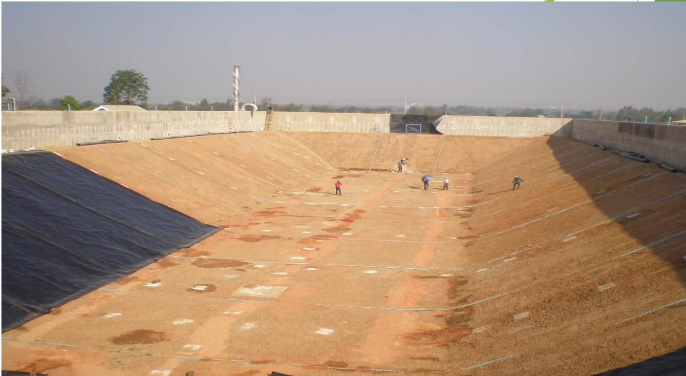
Construction of the reactor
