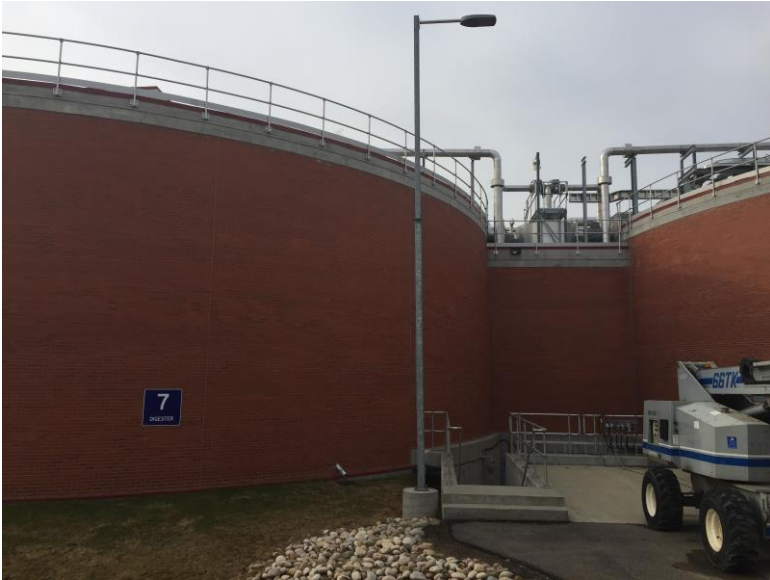
Figure 15 - Digesters 7 & 8 that will be converted from mesophilic to thermophilic operation
