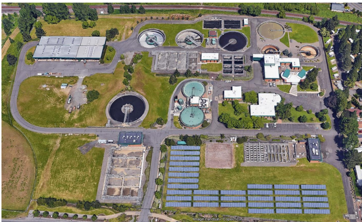
Figure 21 Aerial of Gresham Wastewater Treatment Plant
