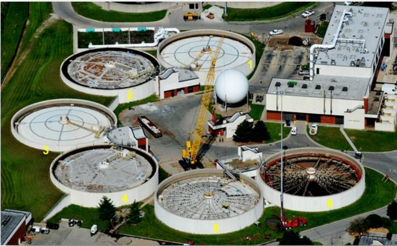
Figure 19 – Digesters at the Des Moines Water Reclamation Facility
