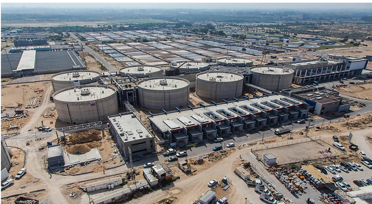
Figure 8 – Aerial of Shafdan Anaerobic Digestion and Cogeneration Facility
