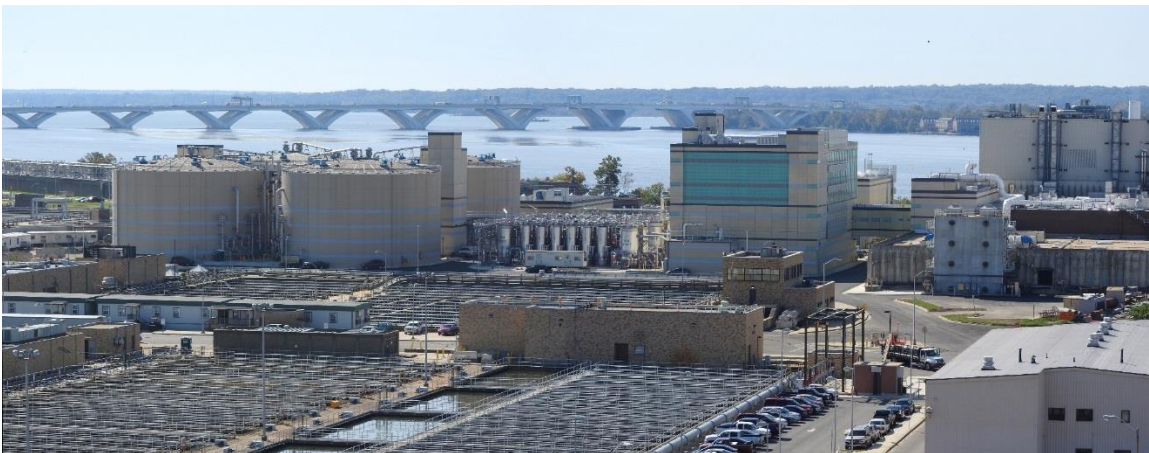
Figure 16 – Thermal Hydrolysis Process and Anaerobic Digestion Facility
